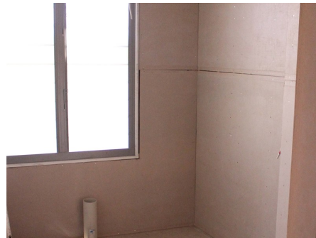
Fibre Cement Sheeting To Bathroom & Ensuite
